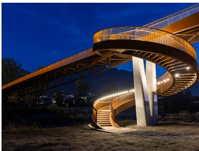
LaneLED WALL, Passerelle de Torretta Bellinzona
